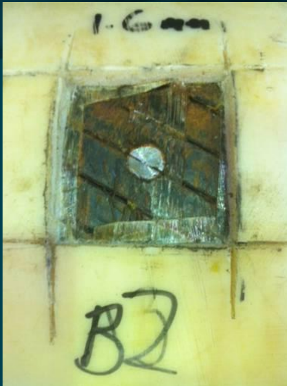
Metal loss defect
