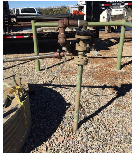
Figure 5 (right). Standpipe, plumbed to temporary receiver tanks
