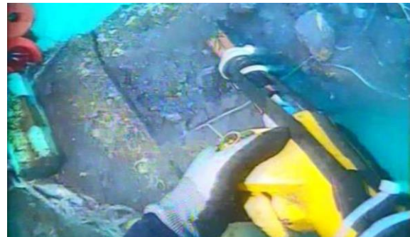
Figure 2: Removal of concrete coating
