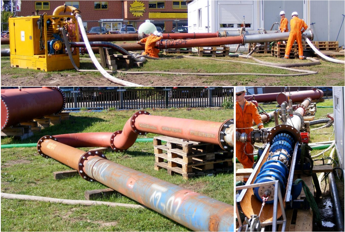
Figure 6-8: Pump test executed in 2013
