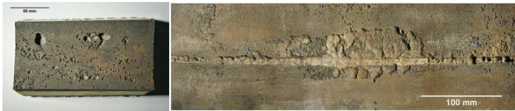
Figure 16-17: Pitting corrosion (left) and girth weld corrosion (right)
