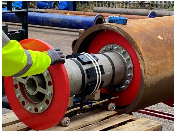
Figure 5: Test pig being inserted into the pipe
